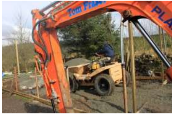
Work at Tinnisburn
